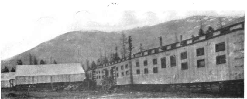
Modern lumber camp on cars, Humbird Lumber Company, Idaho. The cars are equipped with electric lights, shower baths, laundry, and dry room. Twelve men to one car. Spring beds, clean sheets and blankets are supplied.
