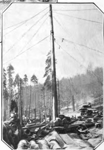
At its destination, the tree, firmly "planted," served as a lead pole for pulling and loading logs at the terminus of the logging road.
