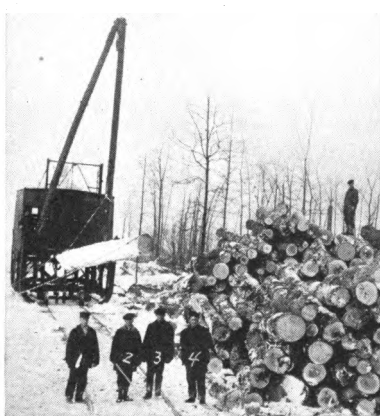
One of Company's Steam Loaders
